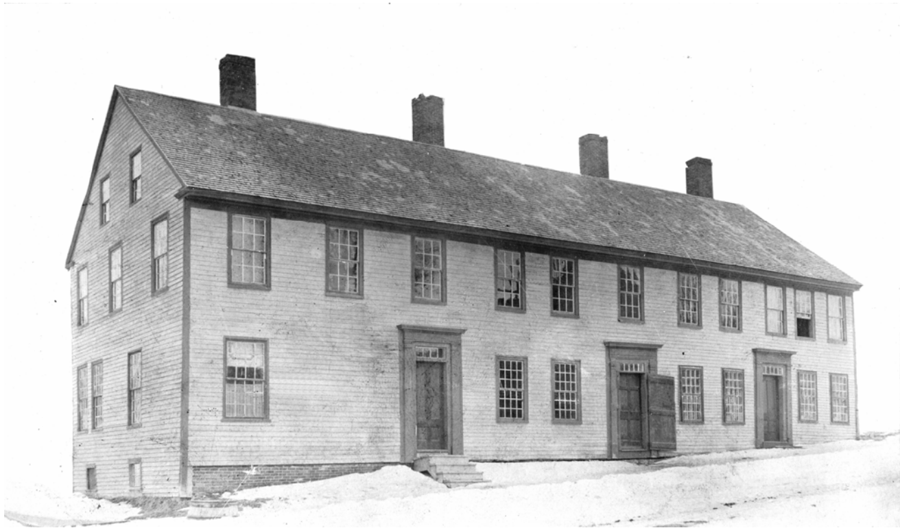
The Mullet Block, was located on the corner of Main and Perkins Streets. Wheeler states that during the British occupation (1814 -1815) the officers of the 29 th Regiment of His Britannic Majesty held their mess here. This building was torn down between March 17 and 18, 1894, and replaced with what is now the Pentagöet Inn.
