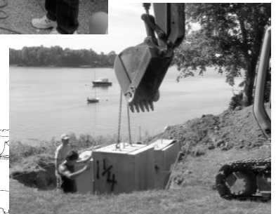
We watched the foundation bases lowered into place.
