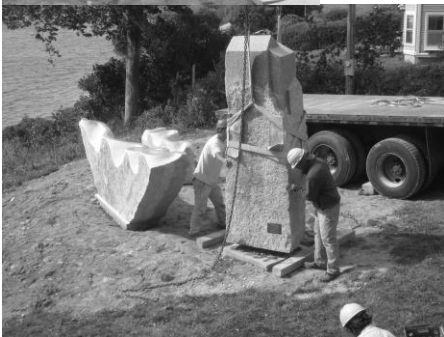
And, finally, the 3 rd stone was set in place.
